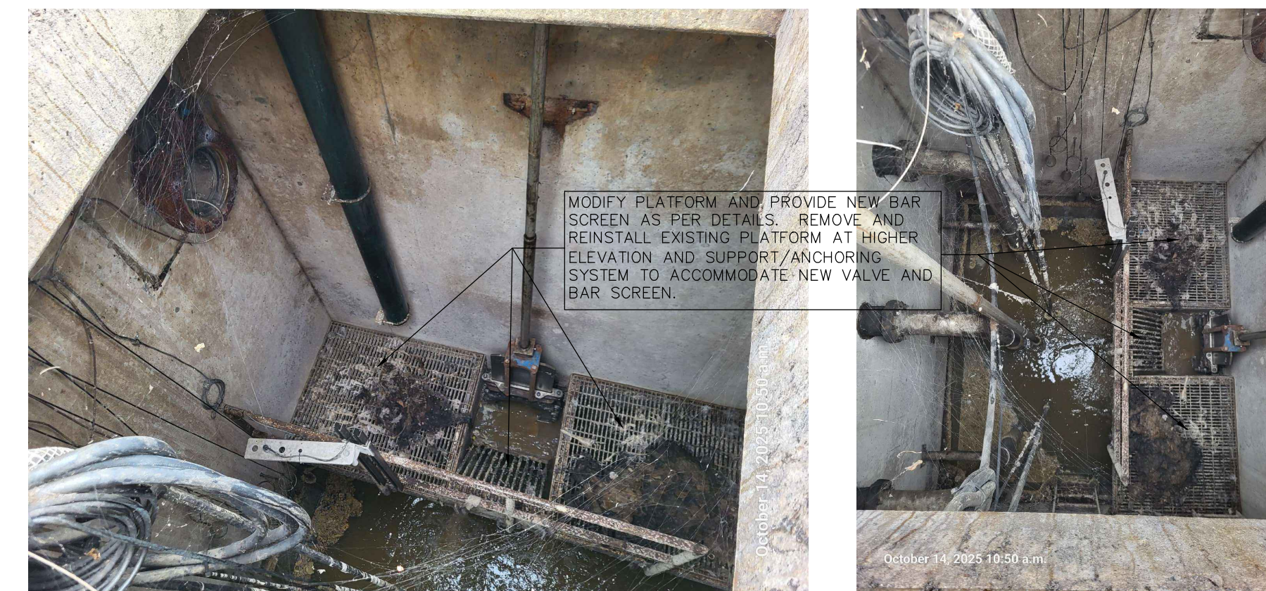
EXISTING WETWELL - BELOW GRADE
